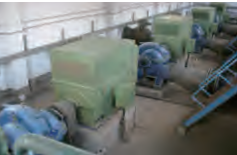
↑ 河北峰峰集团薛村矿电厂 (SLOW 200-530(I)AT,4台) Hebei Fengfeng Group Xue Village Mineral Power Plant
