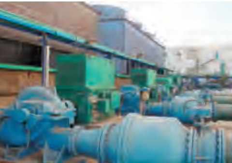
↑ 云南富瑞化工 Yunnan Furui Chemical Industry (SLOW 400-550(I),4台、SLOW 350-520A,5台)
